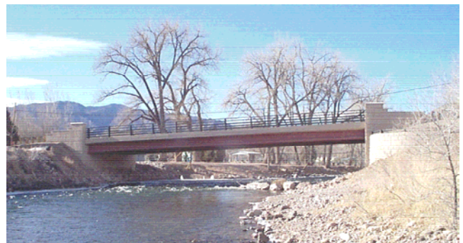
EXISTING FOURTH STREET BRIDGE SITE
